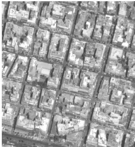
Figure 2. The distribution of daylight differs depending on the type of street grid. The second grid (middle) is a proposal which has especially good access to daylight. The third grid is the darkest but also has the largest variety of form of the urban blocks.
