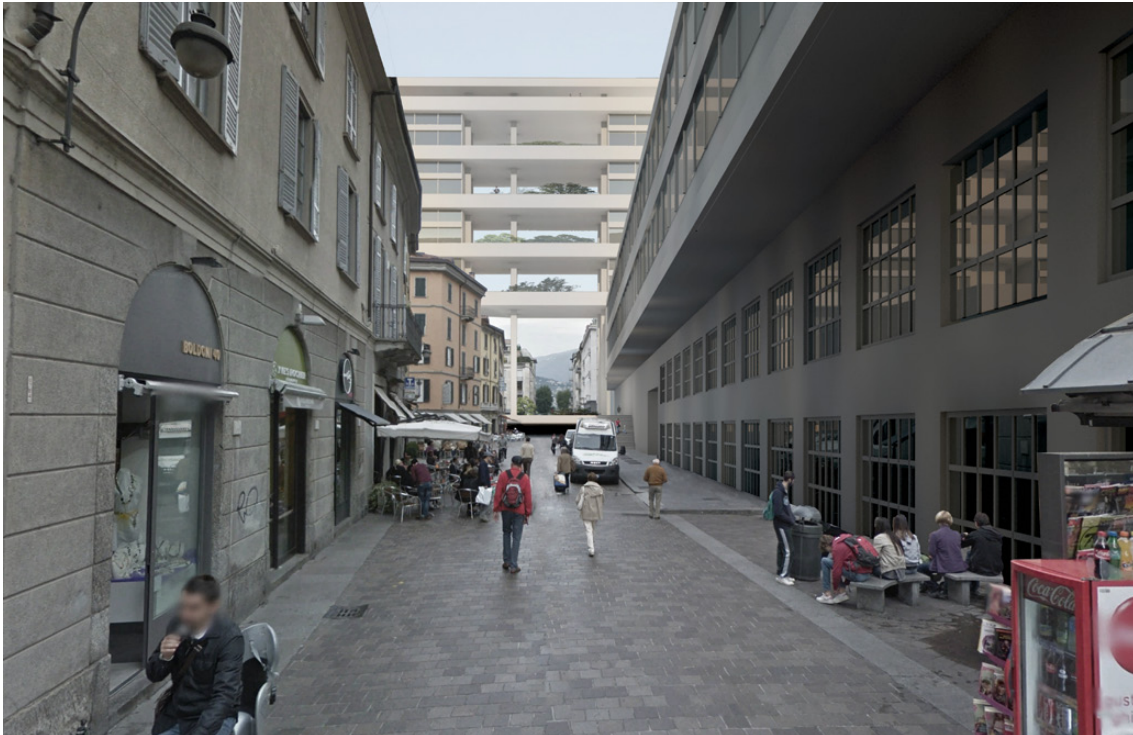
Figure 2. The Cortesella macrostructural building viewed from via Plinio (© Luca Lanini e Brunello Favilla).
