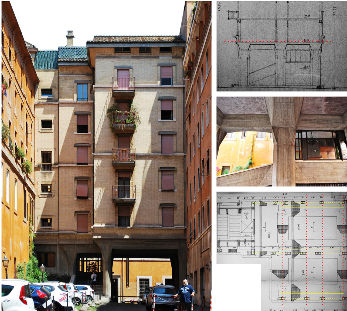
Figure 3. On the left, view of the in-line closing-block building; on the right, section, internal view and structural plan of the concrete “basement”. Elaboration by the author.
