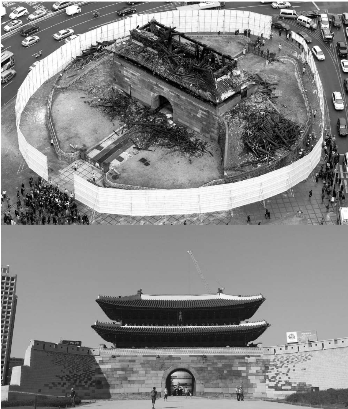
Figure 1. Photograph: Sungnyemun gate, Seoul, Korea; fire (top), reconstruction (bottom). (Source: thehistoryblog.com/archives/25008 , author)
