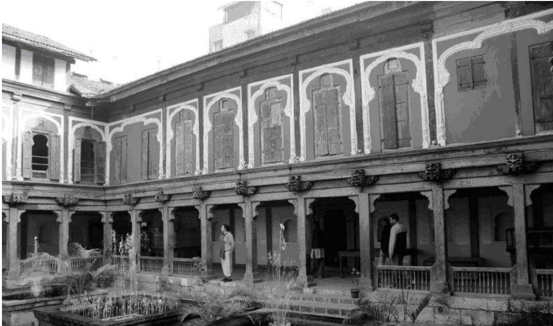
Figure 3. Wada of Pune
