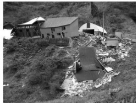
building fell into cliff
