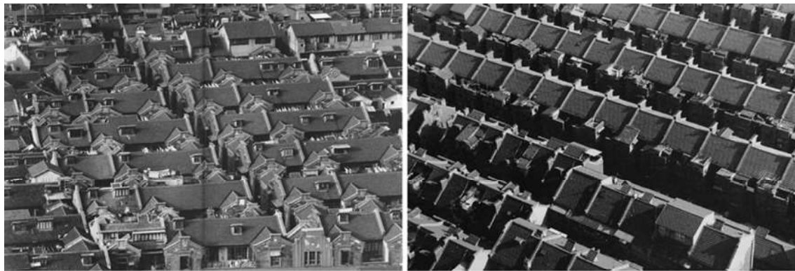
Rooftop scene of a Linong area. (Source: Luo Xiaowei and Wu Jiang,1997)
