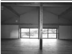
image of the unfinished floor
