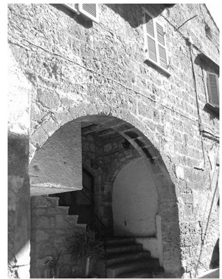
Fig. 21 - Arcaded house with single fornix in via del Duomo in Tivoli (a) and arcaded house with single fornix in Barbarano Romano (b). Sources: pictures and drawing of the authors.
