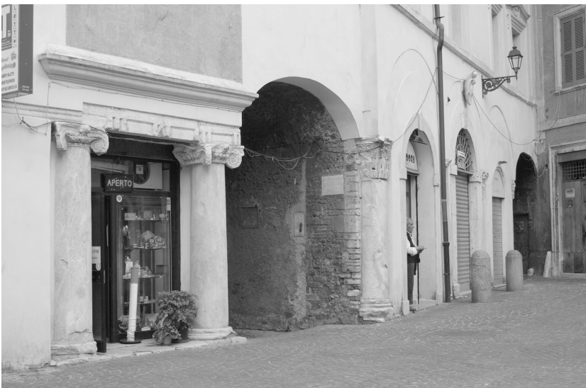
Fig. 24c - Arcaded merged houses with reclaimed elements in Piazza Palatina. Sources: picture of the authors.
