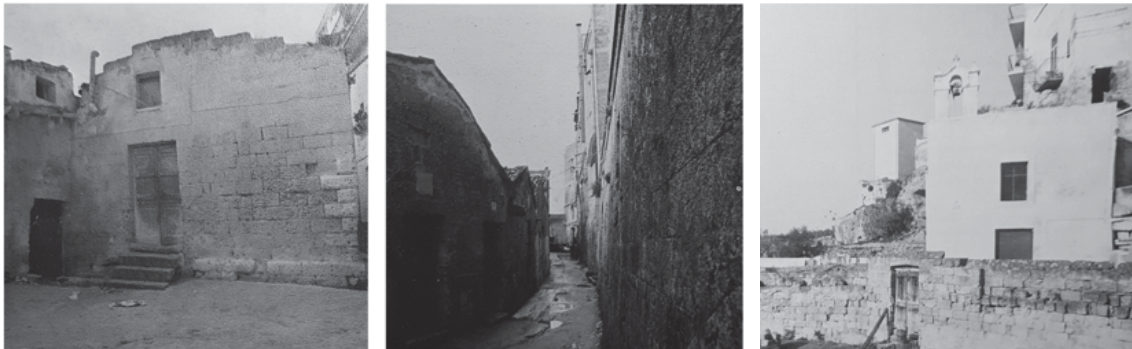
Figure 5. S. Lucia church derives from the "casedda" basic type. The specialised building has the same planimetry and facade of the basic type with bigger dimensions.
