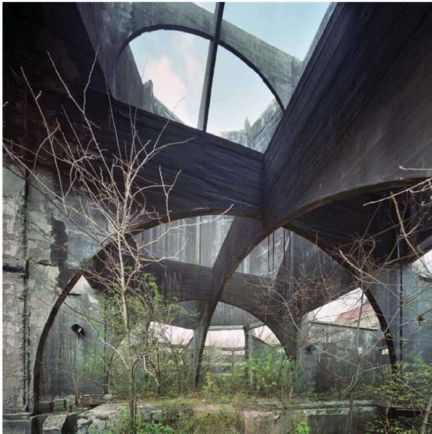
Figure 4. The cooling tower of the West Power Plant, from the 1930's. Photo: Yves Marchand and Romain Meffre.
