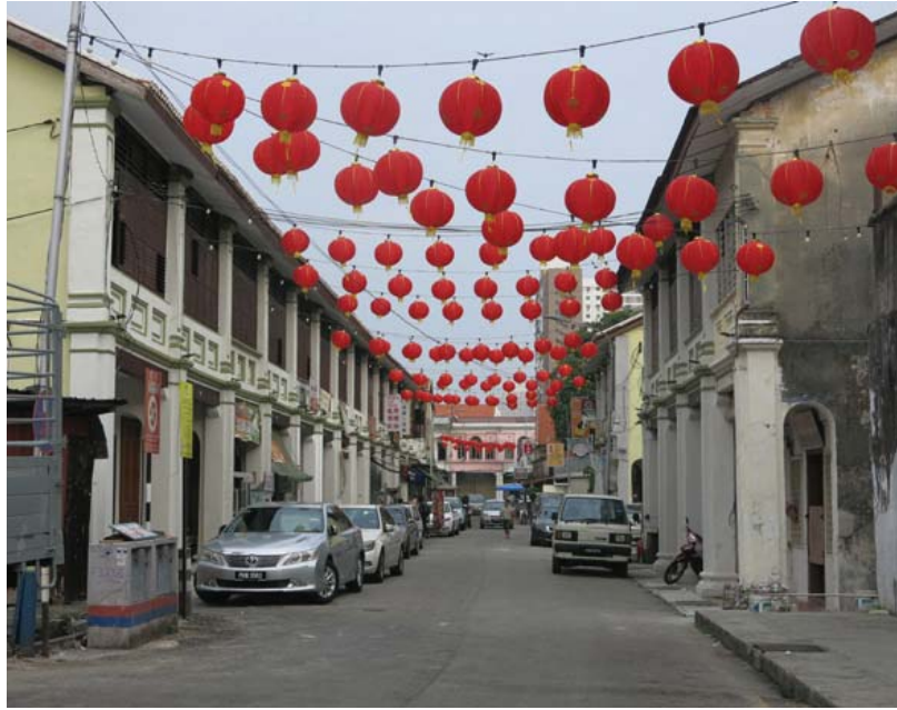
Figure 3. Street view of "Chendol Street", the study site for the Old Cities, New Challenges course, showing the prevalent building type of shophouses.
