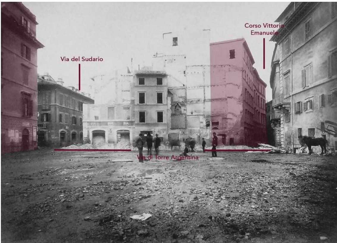
Figure 2. Rome 1885. Urban demolitions for the construction of Corso Vittorio Emanuele and Largo di Torre Argentina. In red the buildings destroyed in the later years.
