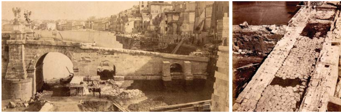
Figure 15. The ramp of Pons Aelius (Ponte S. Angelo) being demolished during the construction works for the Tevere's embankment, 1890 ca.
